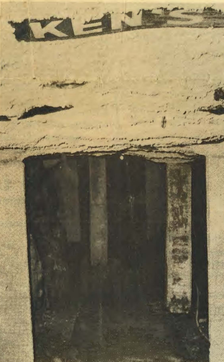
An underground tunnel links the Don Q Inn Best Western Motel to the dining area.
